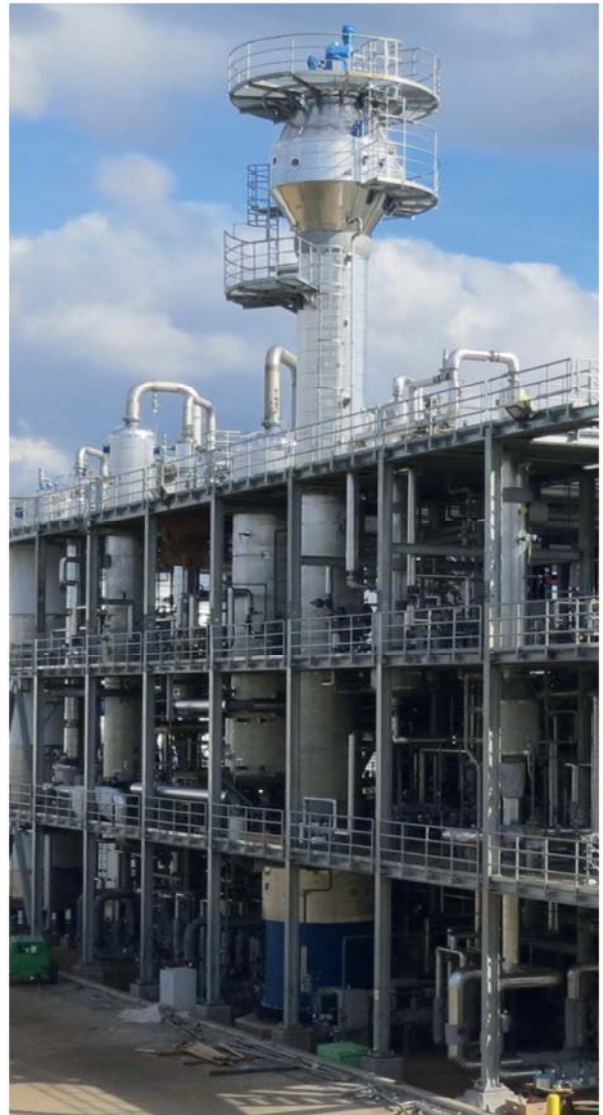
Oil recycling/ diameter decanter \varnothing 3m / height 26m
